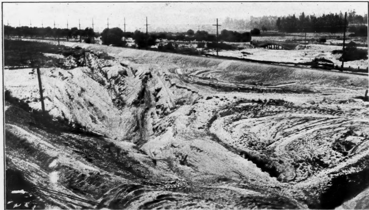
Sand Pit Filled by Flood. Material had been taken from this pit to a depth of about 40 feet. Railroad track south of pit was washed out entirely
